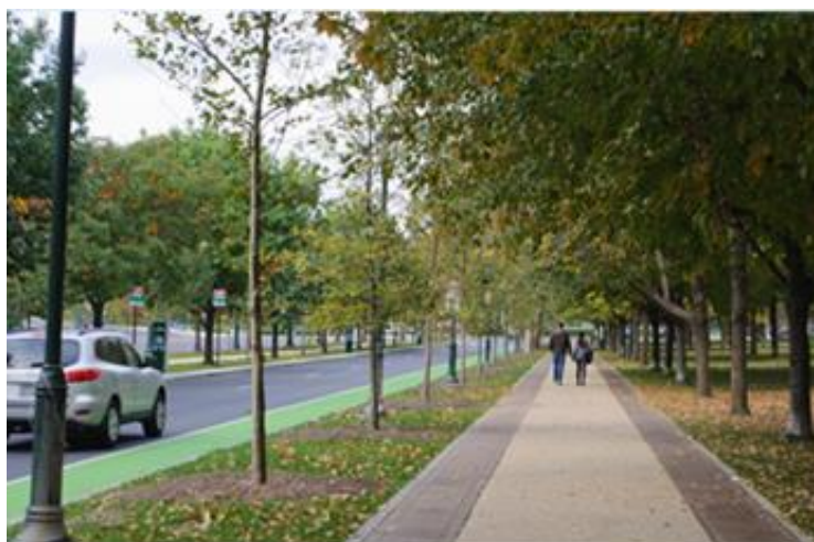
Figure 1: Upgraded local street for revitalization of urban area
